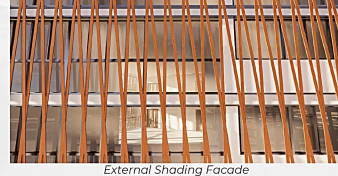
External Shading Facade
